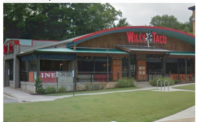
Facade Improvement After
