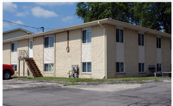
Facade Improvement After
