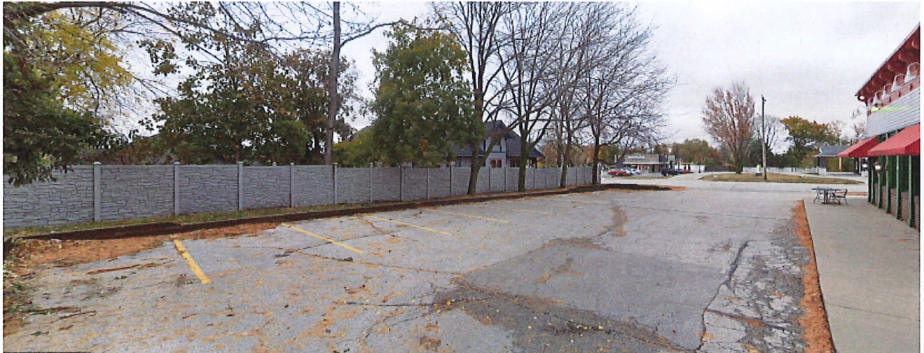
Screening along the north side of the subject property
