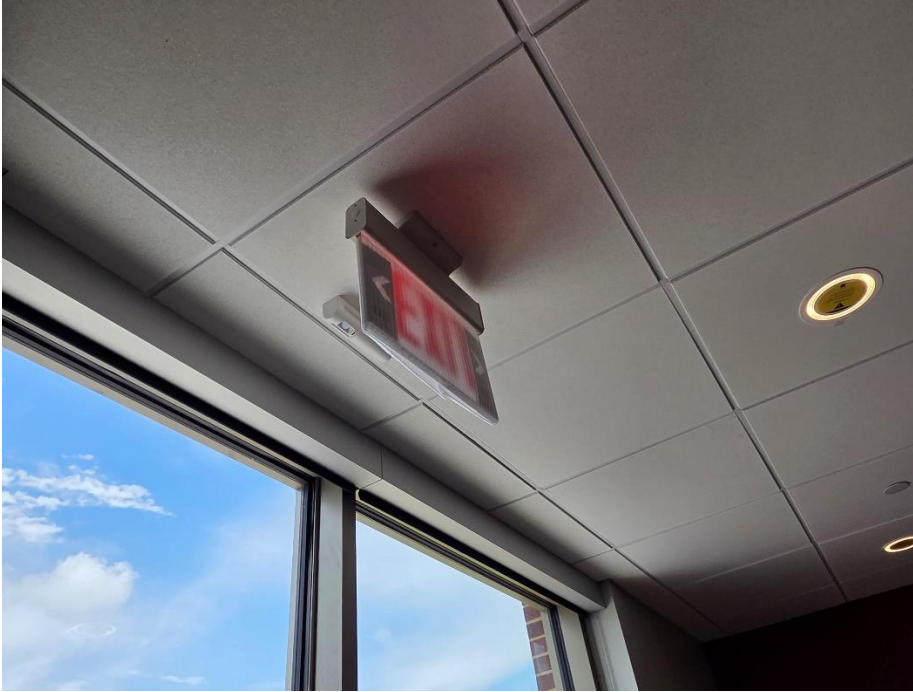
Photo #3 – Missing cover plate
