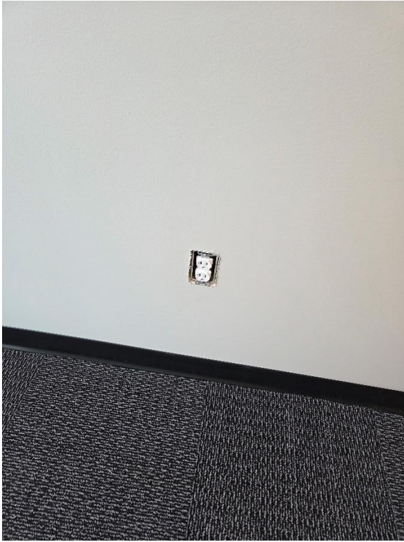
Photo #5 – Cover plates not flush
