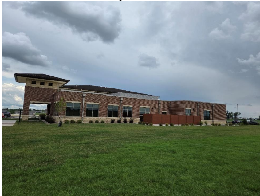
Photo #1 – North Side of Building
