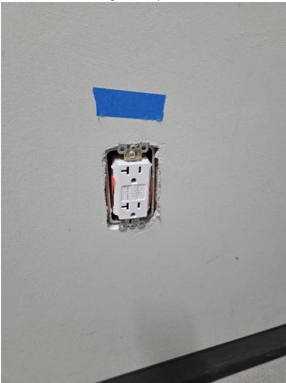
Photo #3 – Missing cover plate
