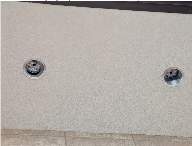
Photo #11 – Signage lights not aimed correctly
