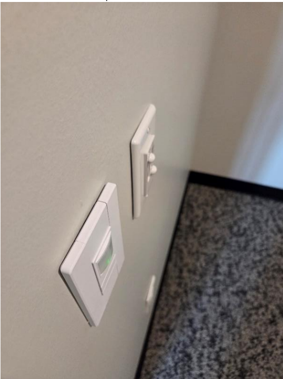
Photo #5 – Cover plates not flush
