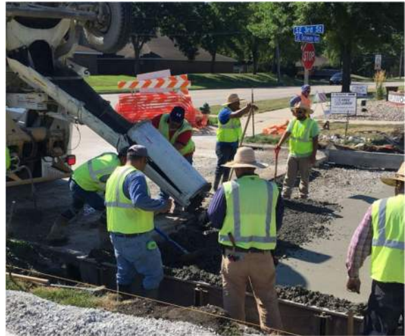
Figure 24 - C-SUD Mixture Placement
