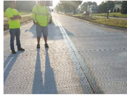
Figure 26 - Longitudinal Joint After Application of a Penetrating Sealer
