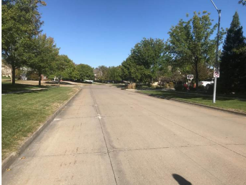
Figure 21 - Joint Shadowing (NE Trilein Drive, North of NE 18th Street)
