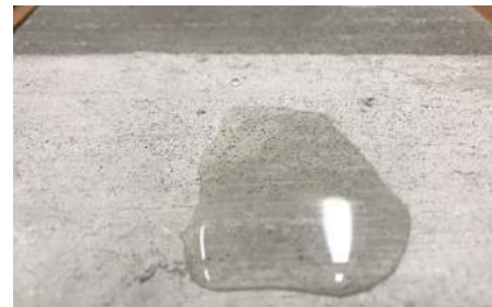
Figure 25 - Water Beading on Concrete Treated with Penetrating Sealer
