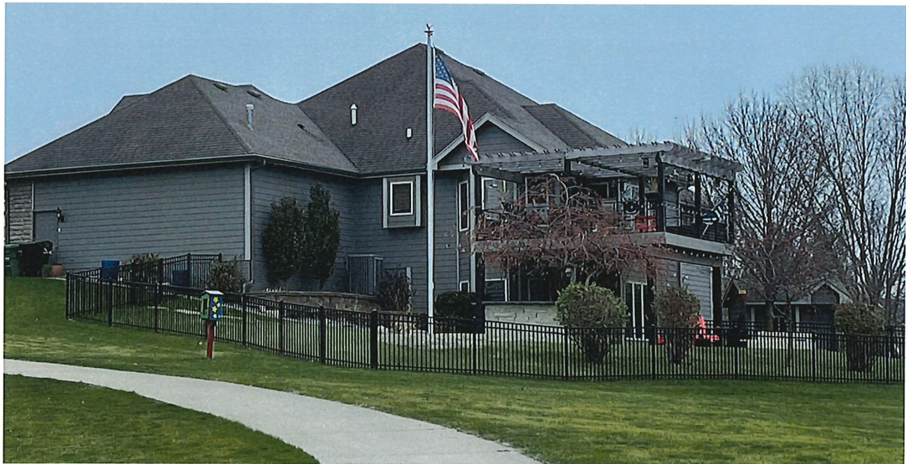
Subject property with existing pergola.
