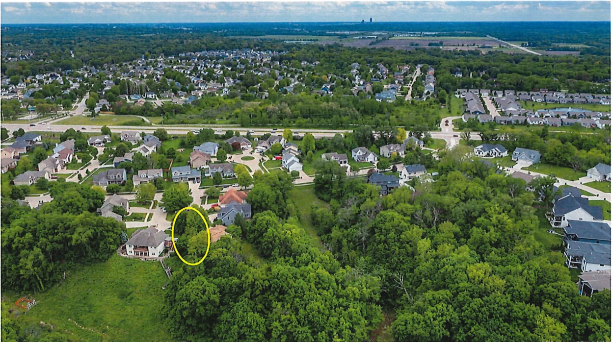
Area to be remedied – view from rear looking south.
