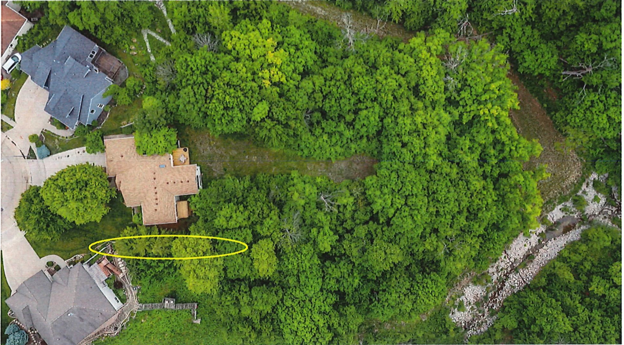
Area to be remedied – view from above.
