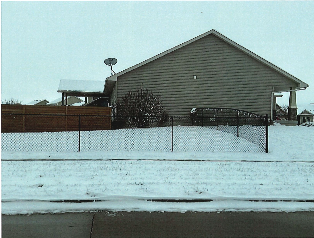
View of the existing covered deck from the south
