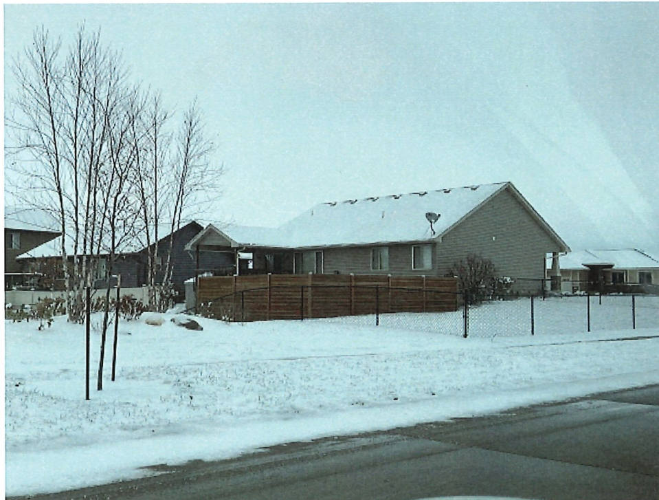
View of the existing covered deck from the southwest
