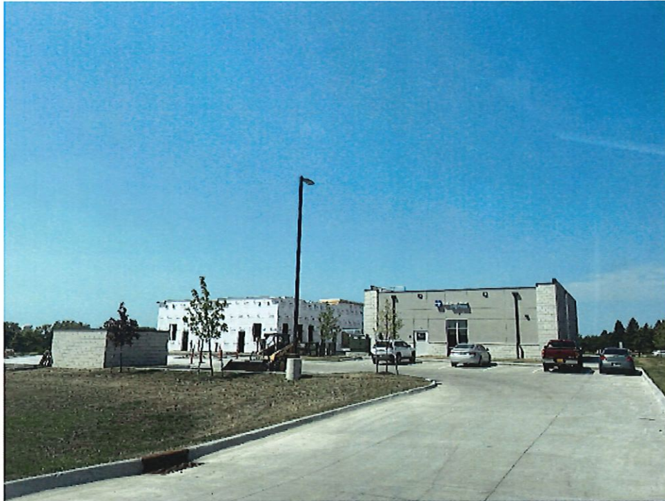
View of 1055 & 1075 SW Orallabor Road from the south
