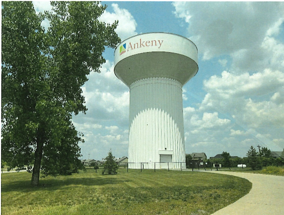
Existing Water Tower at 1841 SW Irvinedale Drive
