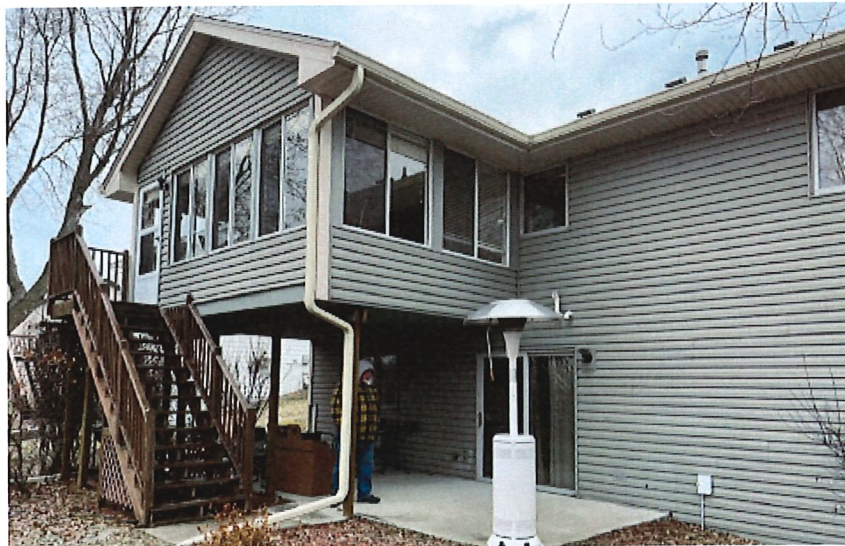
View of the existing sunroom from the NE
