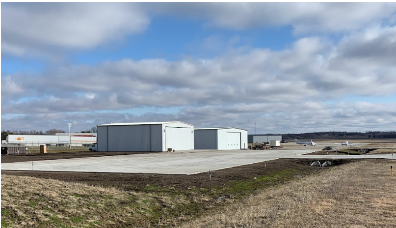
Taxiway D Box Hangar Development
