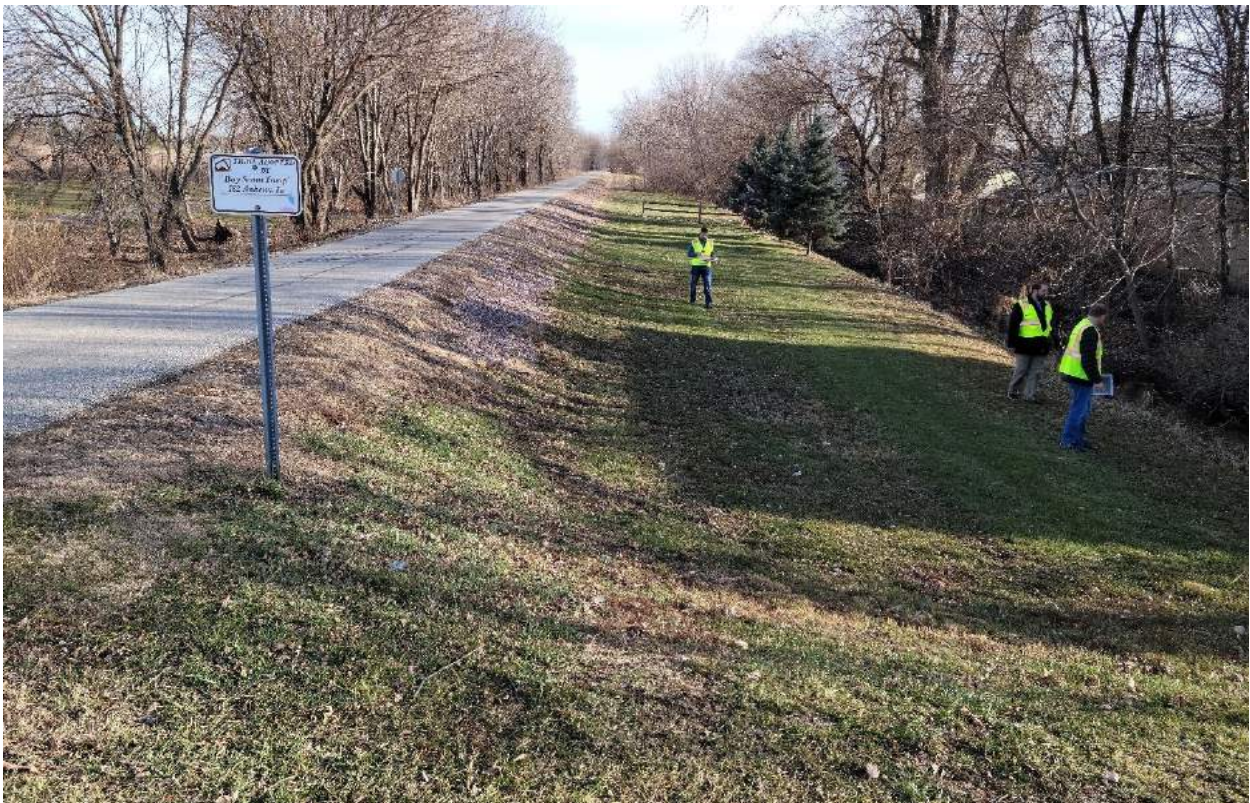
2020-12-04_SurveyWalk_1007 NW State_lookingSE
