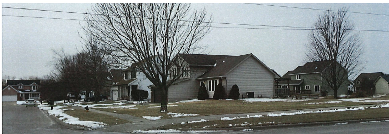
Looking southwest towards the subject property from the north side of NE 18 th Street.
