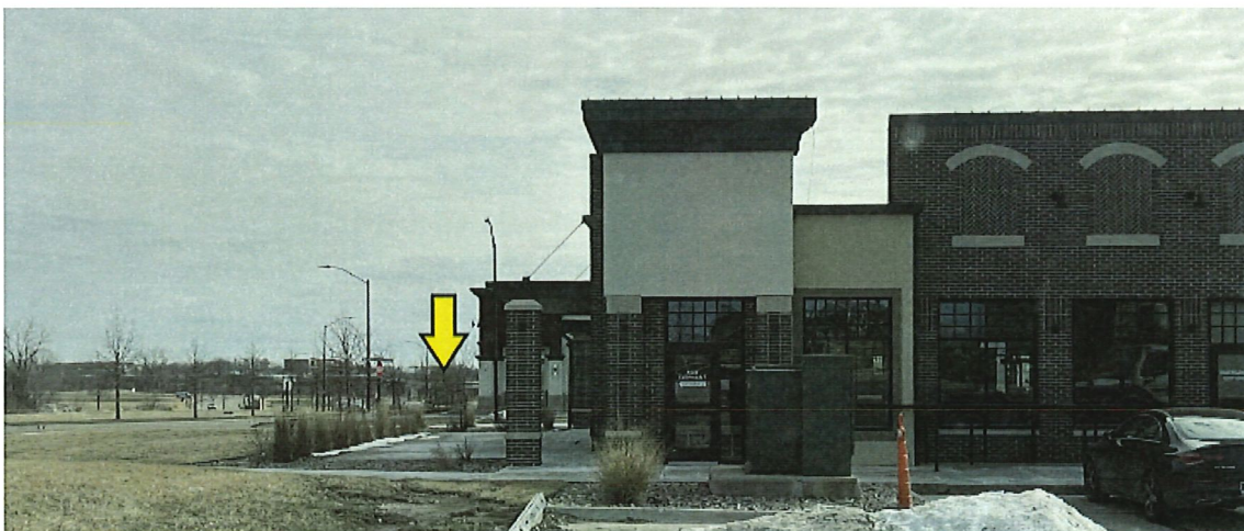
View of the Silk Elephant from the rear parking lot with the arrow pointing towards the service area
