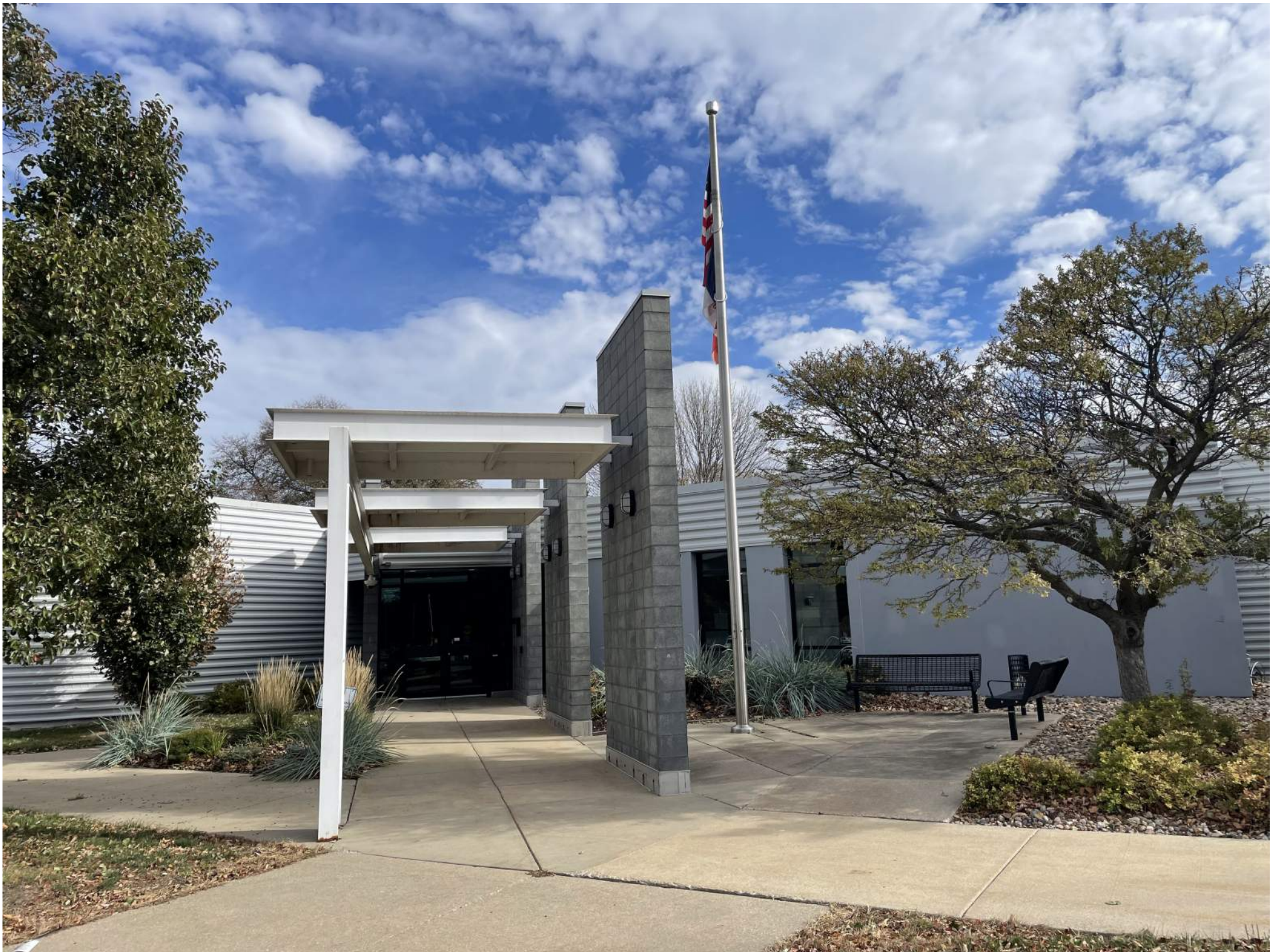
1 PHOTO 1 - ENTRY FEATURE LOOKING NORTHEAST
