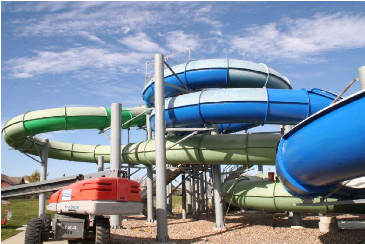
Cascade Falls Gel Coating in progress
