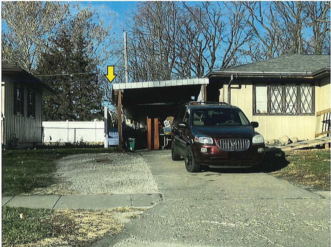
View of the carport visible from SW 2 nd Street. Arrow pointing towards the space between the carport and the neighboring fence.
