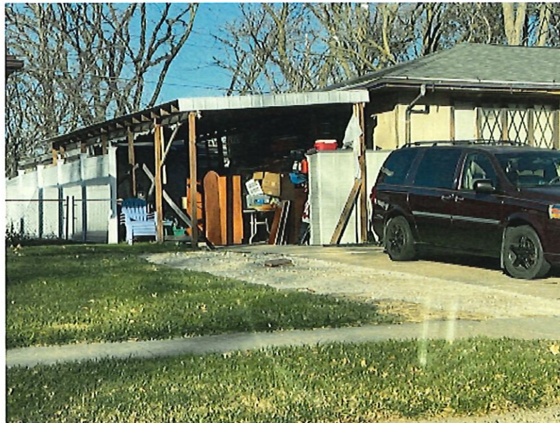
View of the carport visible from SW 2 nd Street
