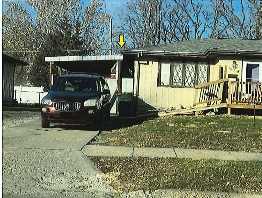
View of the carport visible from SW 2 nd Street. Arrow pointing towards the distance between the carport and the primary structure on the property.
