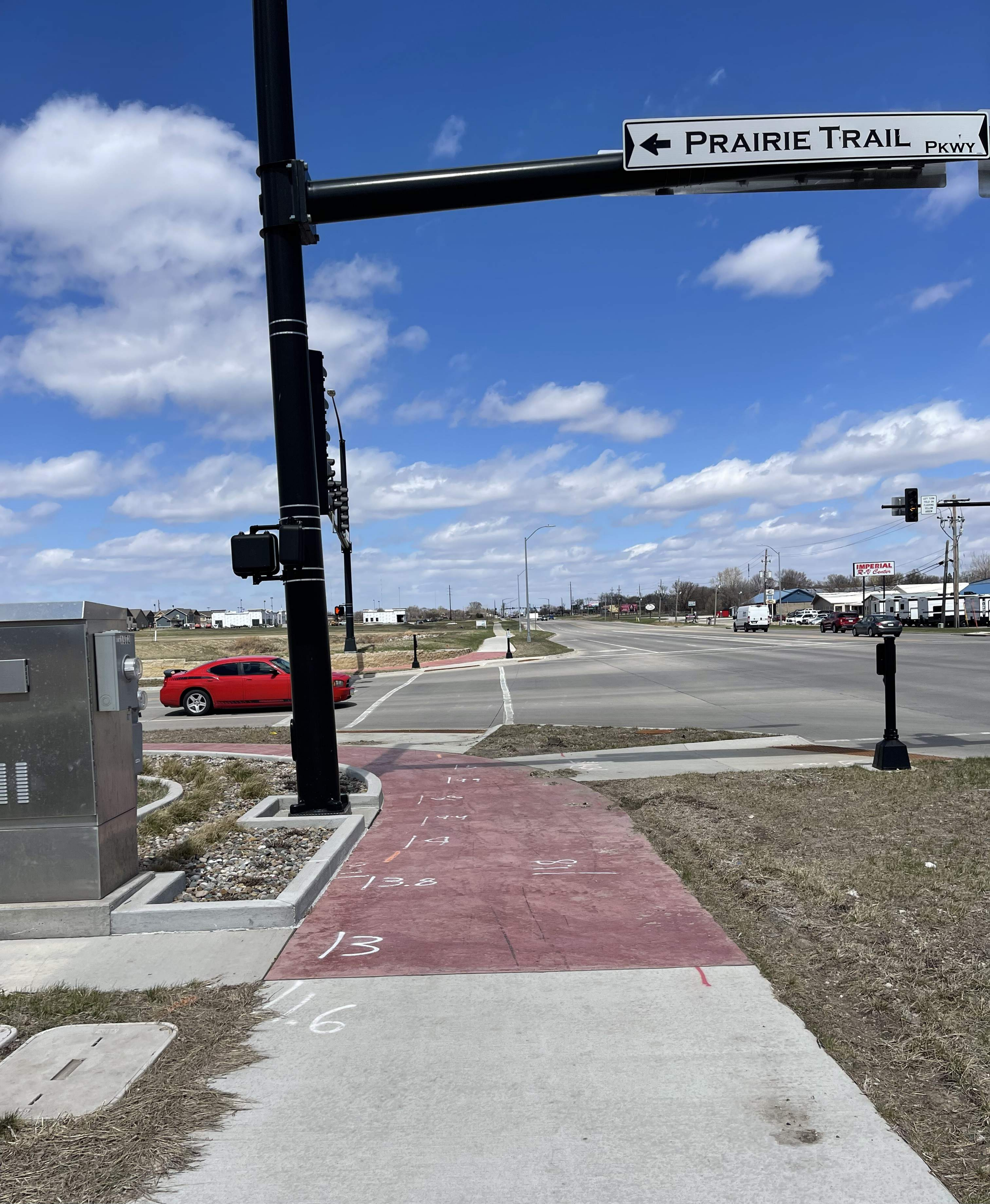
SW Corner of Prairie Trail Pkwy and S Ankeny Blvd - Looking North
