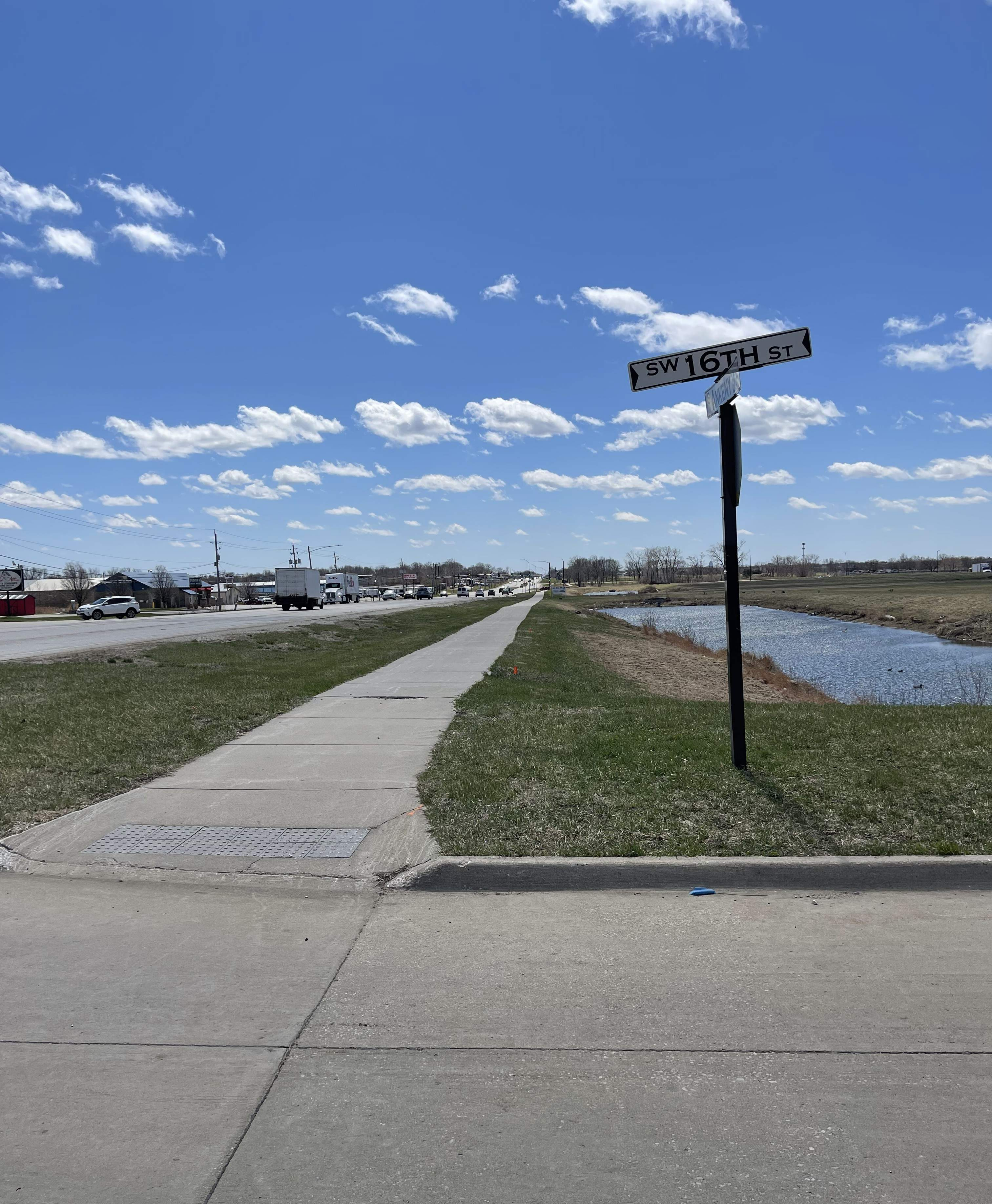
NW Corner of SW 16th St and S Ankeny Blvd - Looking South
